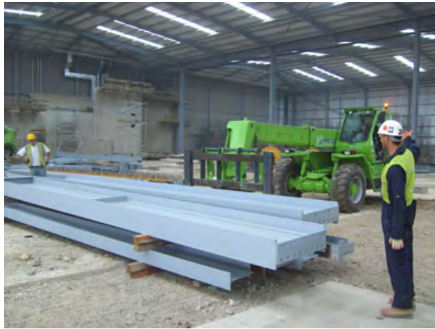
Figure 14 - Use of Wider Fork Carriage
